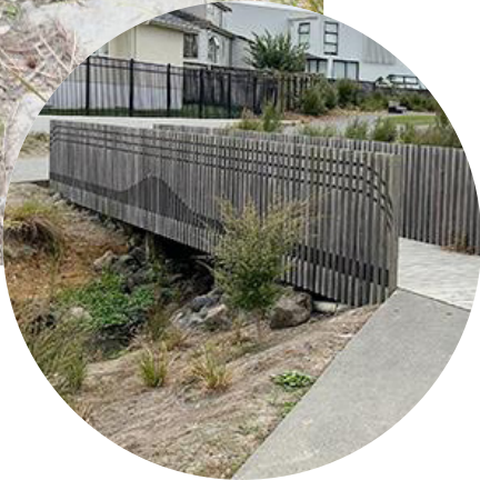
Shared Bridge over stream Provides improved accessibility and safe crossings over streams, roads or difficult terrain.
