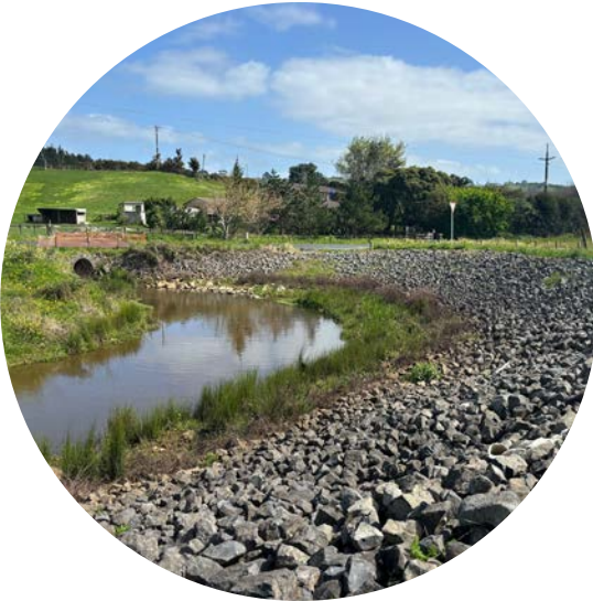
Looking towards Munro Road at the diverted stream along southern edge of the park, featuring rip rap banks
